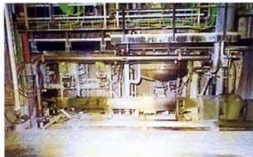
Application: coating kitchen. One VFD-controlled seepex pump N 240-12 with dry running protection TSE 120 and flushing connection. Product: coating color, flow rate: 17 - 182 m 3 /h (75 - 800 gpm), speed: 25 - 245 rpm, pressure: 4 - 8 bar (60 - 120 psi), temperature: 20 - 55° C, spec. gravity: 1.6, solids content: 60 - 70% wt, viscosity: 3500 - 5000 cps
