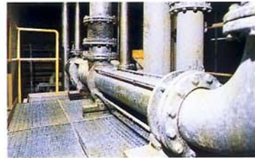
Application: water and waste water recycling in a paper machine. One VFD-controlled seepex pump BN 202-6L with flushing connection and dry running protection
