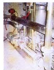
Application: coating kitchen. seepex pumps BN 70-6L with dry running protection TSE 120 and single-acting mechanical seal. Product: coating,
