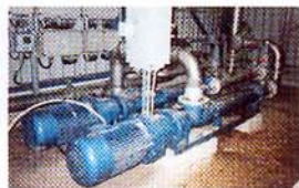
Juice Thickening Two seepex pumps BN 70-12, product: syrup from thickening to crystallization, flow: 70 m 3 /h / 308 usgpm, speed: 370 rpm, pressure: 11 bar / 156 psig, temperature: 15° C / 59° F, viscosity: 822 mPas, SG: 1.37 kg/dm 3
