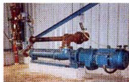
Crystallization A seepex pump BN 35-12, product: thick juice, flow: 25 m 3 /h / 110 usgpm, speed: 300 rpm, pressure: 10.3 bar / 146 psig, temperature: 15° C / 59° F, viscosity: 822 mPas, SG: 1.37 kg/dm 3
