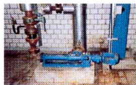
Crystallization seepex pump BN 17-6L, product: 'A' sugar run off, flow: 13 m 3 /h / 57 usgpm, speed: 265 rpm, pressure: 2.66 bar / 38 psig, temperature: 50° C / 122° F, viscosity: 200 mPas, SG: 1.4 kg/dm 3
